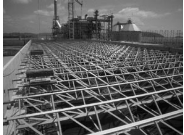
Photo 1 Λ Truss System for RDF plant building
